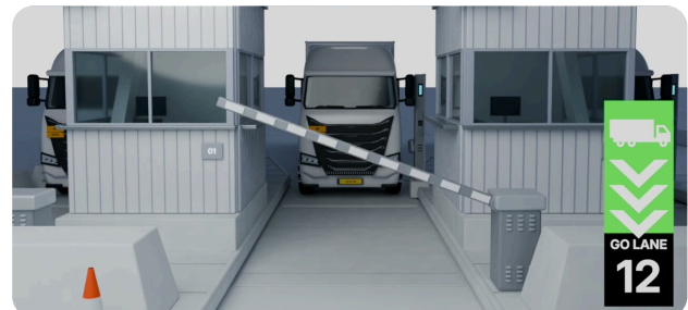
FIGURE 2 The port's check-in system clears the booking. Its sign shows the lane and its barrier opens.
