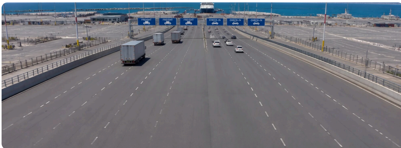
FIGURE 1 The approach road is where the record starts. Lane signage and gantry by the port.
